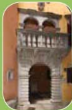
Franchovich palace Franchovich-Palast
